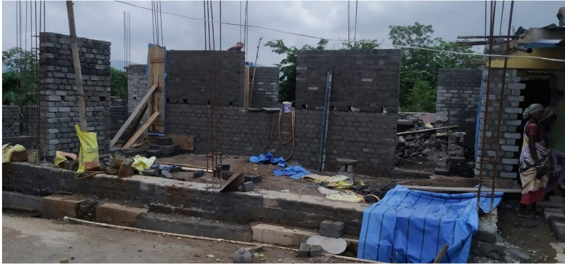
Figure 6: Ongoing Kitchen Construction
