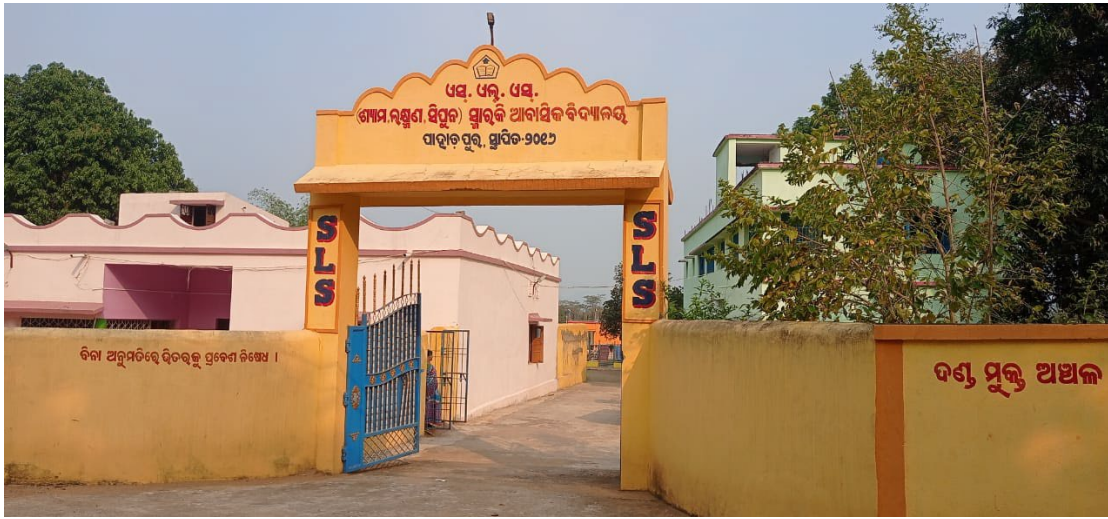
Figure 2: Completed Compound Wall and Entrance
