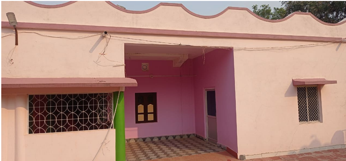
Figure 4: Existing Dormitory Facility
